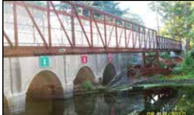
TEMPORARY/PERMANENT PEDESTRIAN BRIDGE, 8' X 240' MANUFACTURED, ENGINEERED, BUILT IN 2011, 120' CLEAR SPAN. CALL FOR MORE INFORMATION.
